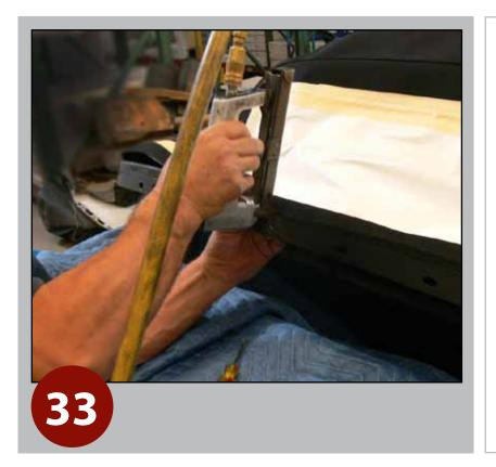
Using your heavy duty stapler or compressed air stapler as shown, begin stapling from the center outward.
